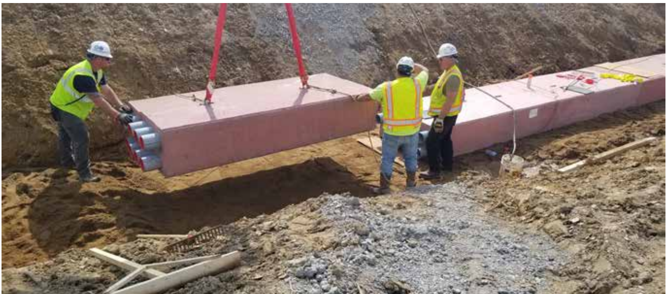
Precast duct bank installation. Source: Forterra.
