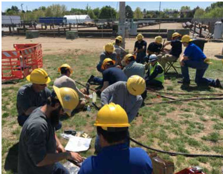
Installation skills training with immediate on-site factory-comparable testing and qualification. Source: IMCORP.
