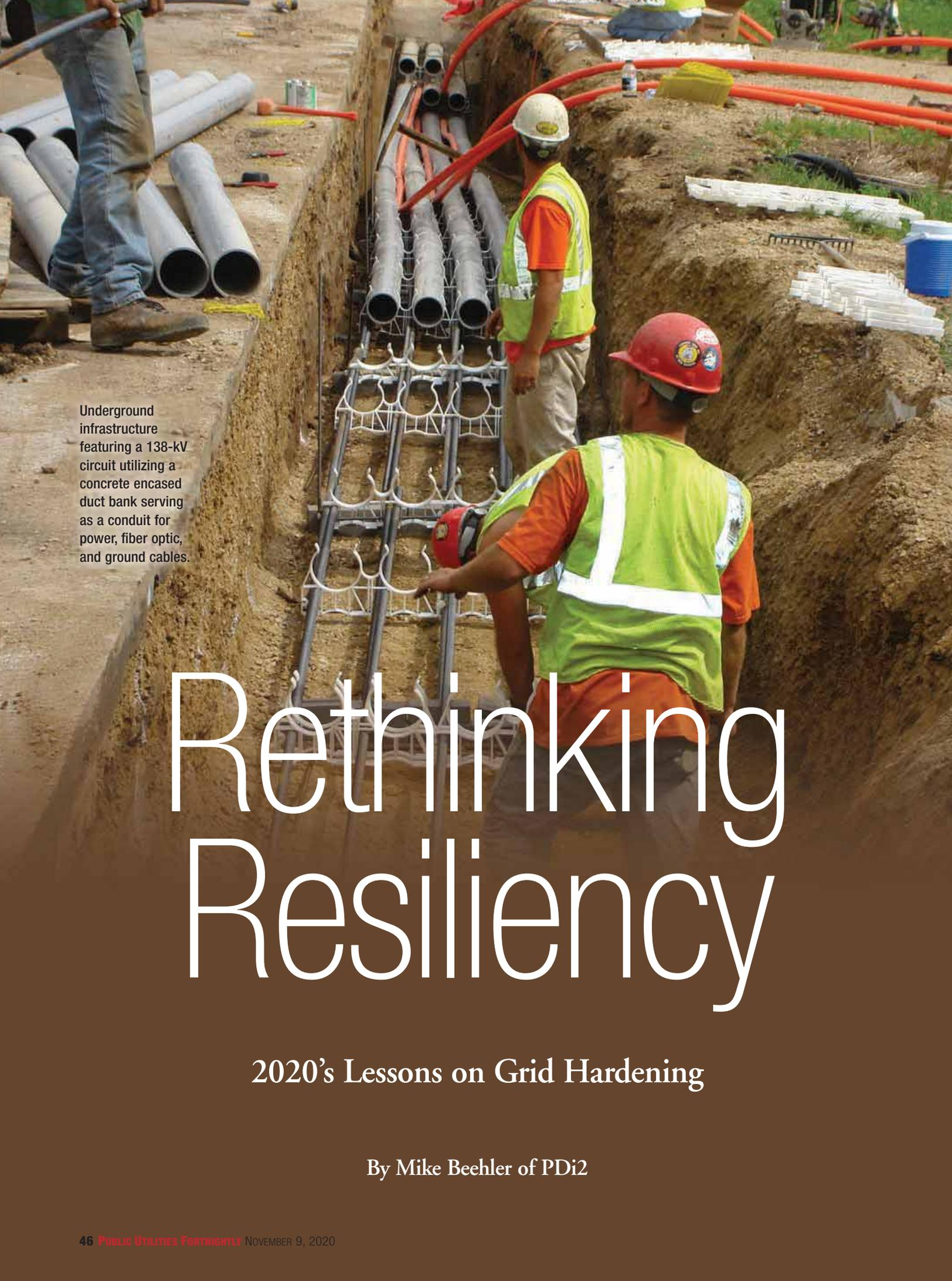
Underground infrastructure featuring a 138-kV circuit utilizing a concrete-encased duct bank serving as a conduit for power, fiber optic, and ground cables.
